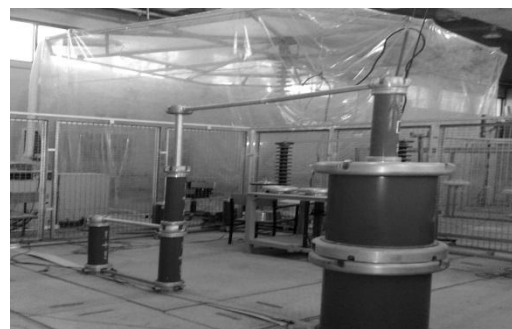
Fig. 1. Experimental setup: power supply, CVD and fog chamber.
